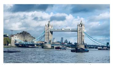
opens to allow tall river vessels through) and a suspension bridge. The bridge itself is two towers, joined at the top by two pedestrian walkways and with a road/pedestrian surface at the base.
